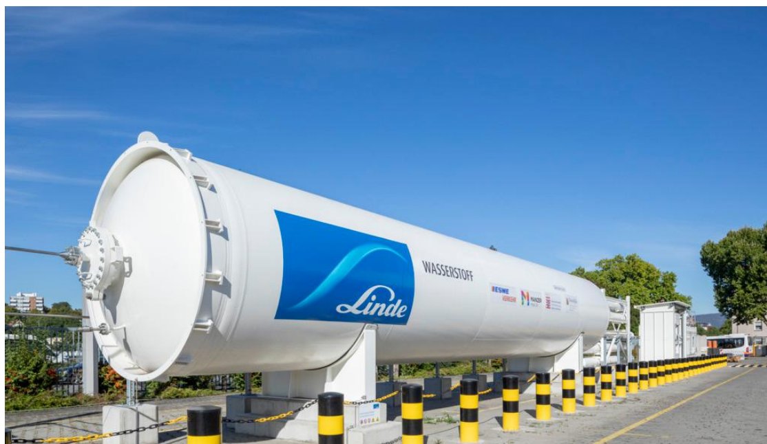
Figure 5.3 A pressurized hydrogen storage tank
