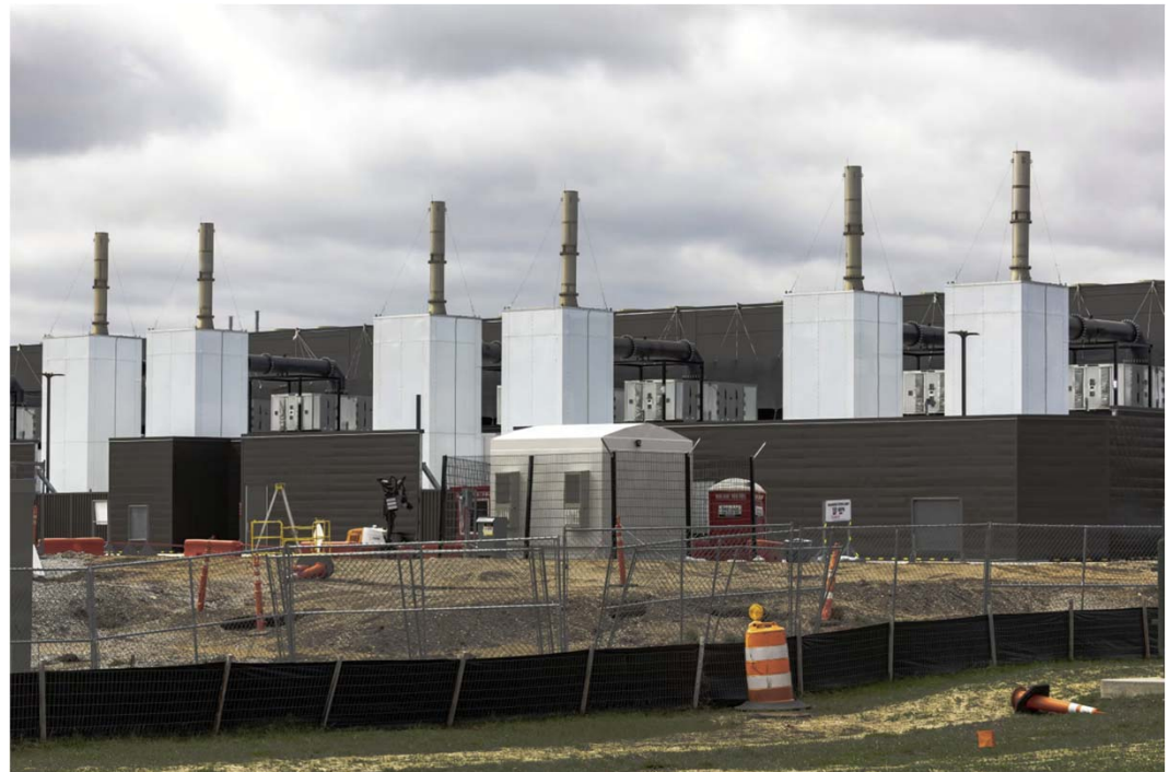
Amazon's data center in New Carlisle, Ind. Jim Vondruska/Reuters
